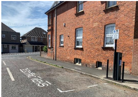
Figure 4: On-street chargepoint installations
