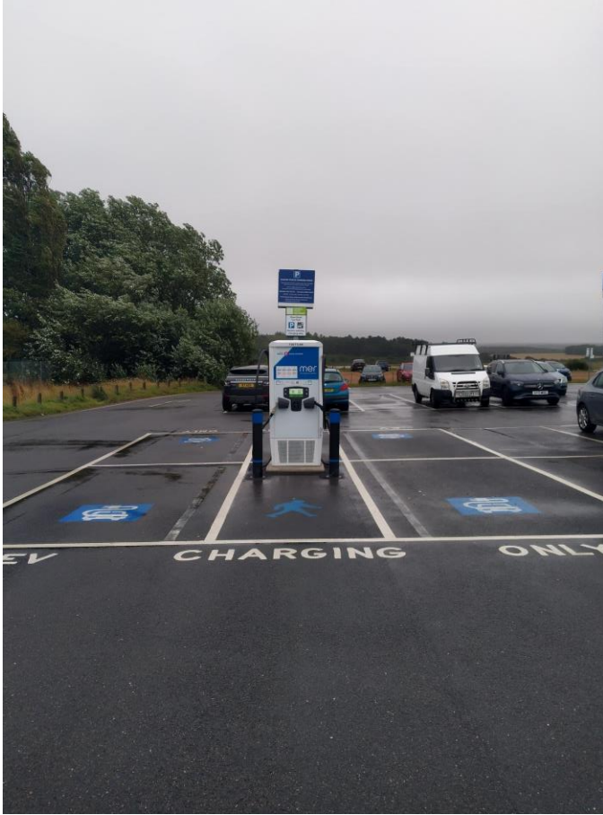
Figure 8: Tritium 50kW rapid chargepoint at River Road car park, Yarmouth. This chargepoint has 1 x CCS connector and 1 x Chademo connector.
