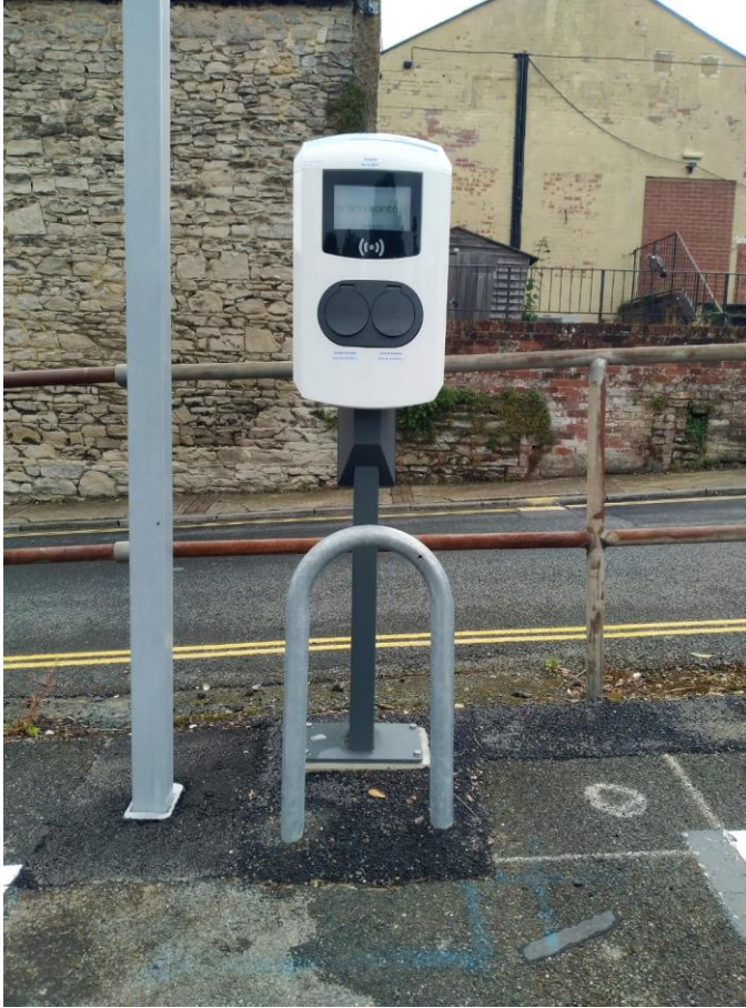
Figure 7: Alfen Eve 22kW chargepoint at St. Thomas' St (upper) car park, Ryde
